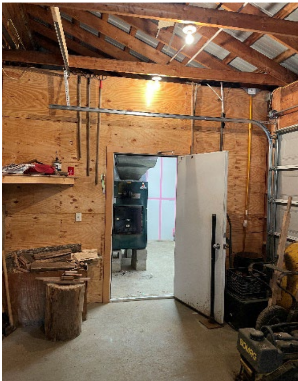
Photo 3: Furnace room separation
