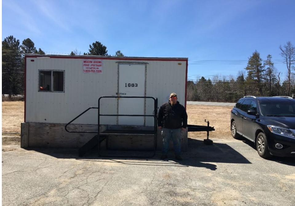
Photo-9: View of temporary construction trailer to house highway maintenance employees during the winter months.
