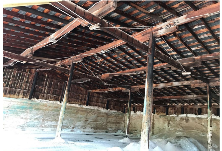
Photo 2 – Lincoln (115) – Salt Shed Internal Structure
