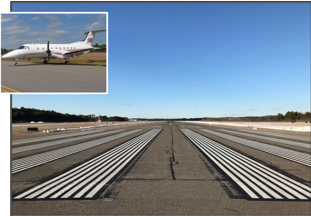
Figure 2: View of Concord Municipal Airport's Runway 17-35.
